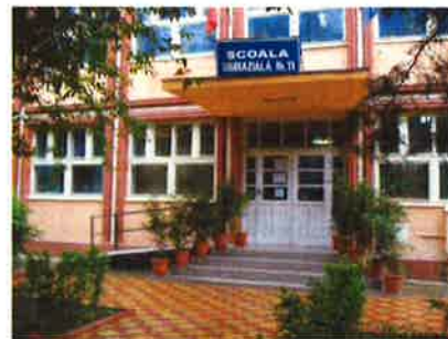
Primary School no. 11 Buzău, Buzău County Source of photo: Andreea Beatrice
